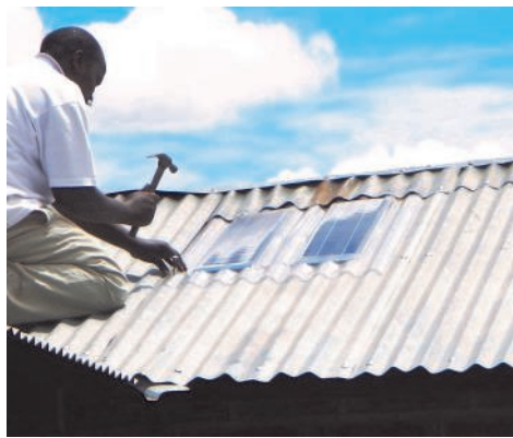
Picture: Solamander 36 Watt Photovoltaic panel mounted on a corrugated roof and held in place with nails
